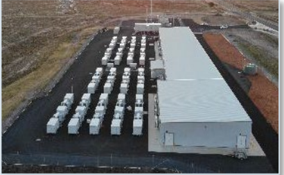
Vena Energy selects Doosan GridTech as EPC for 100MW Wandoan South BESS
