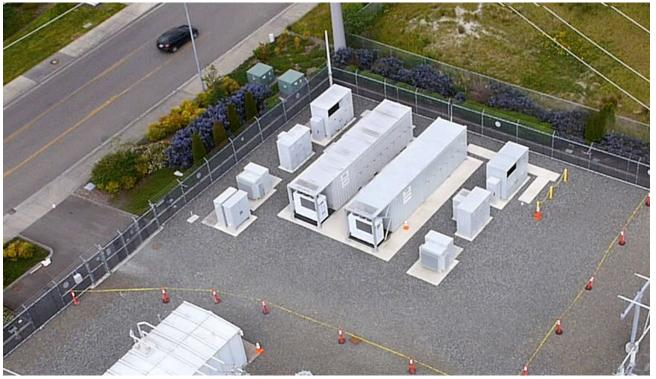
Location: Everett, WA Utility Offtaker: Snohomish County PUD Battery: Mitsubishi, LG Chemical, and UET Inverter: Parker and Siemens Control Software: DG-IC<sup>®</sup> and DG-DERO<sup>®</sup> Open Standards for Energy Storage
